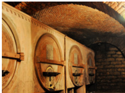
The concrete tanks at Cantine Valpane
